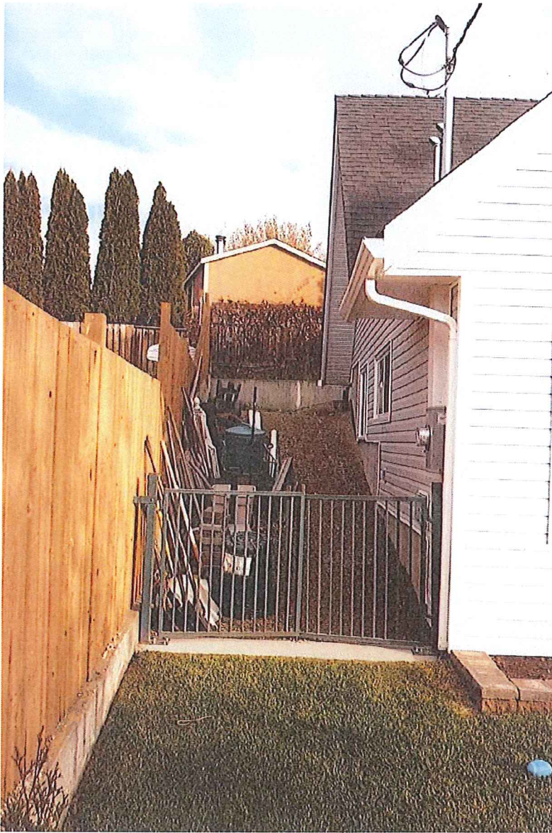
West Side of Accessory Building
